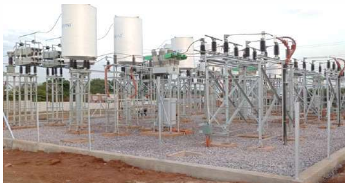
33KV, 27MVAR HT Fixed Outdoor Type Capacitor Bank for 50 MW Solar PV Plant for Indian Railways at Bhilai, Chhattisgarh
