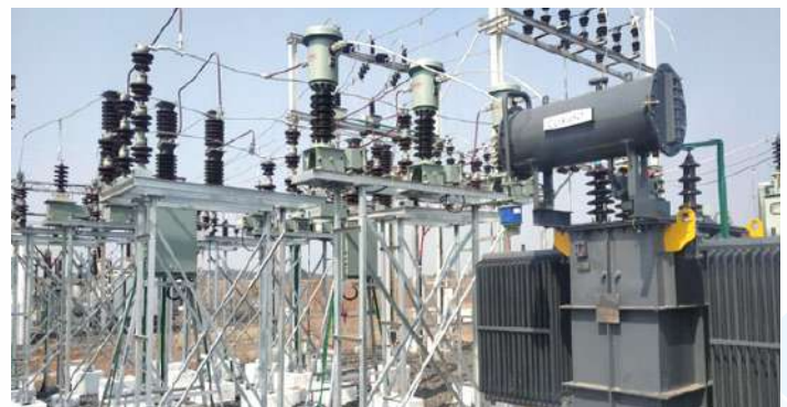
SHUNT REACTOR & STATCOM for Compensation of Transmission Line Capacitance at Malwa Solar Power Generation Pvt Ltd., Kachalia
