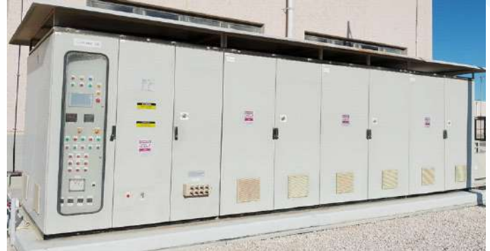
17.5KV MV Automatic Capacitor Banks for Saline Water Conversion Corporation (SWCC) Jubail PS1 Station, Saudi Arabia
