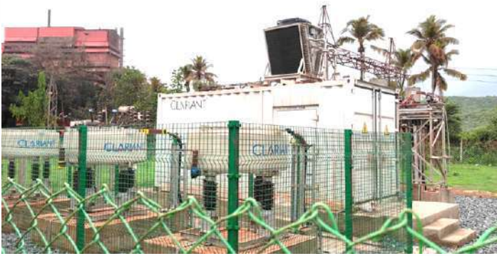
MV STATCOM for Steel Plant of Lloyds Group
