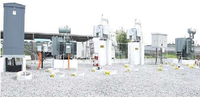
33KV Hybrid Reactive Power Compensation with SVG and Shunt Reactor for APRAAVA Energy (100MW Veltor Solar Plant)
