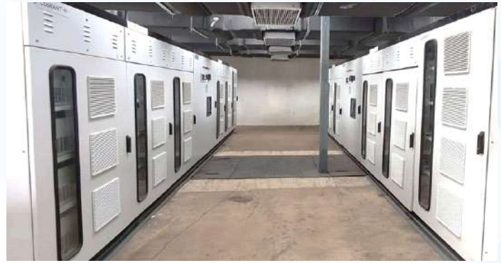
LV SVG/STATCOM for Arc Furnace Plant of BAJAJ GROUP
