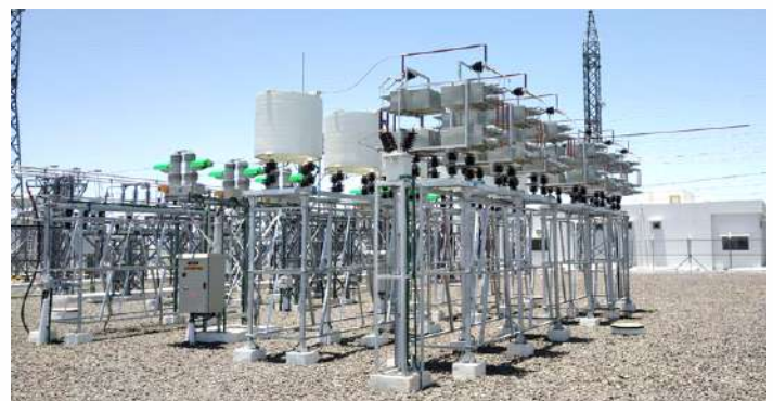
33KV, 17MVAR HT Automatic Outdoor Type Capacitor Banks for Siddhapur Pooling Substation Project, Gujarat
