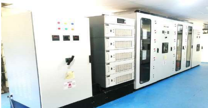
LV & MV SVG/STATCOM with APFC Capacitor Banks for Hindalco Industries Limited, Taloja (ADITYA BIRLA GROUP)
